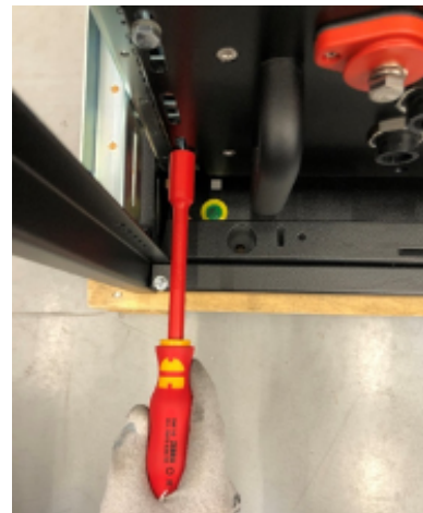
Picture 23 Li.ONESS modules tighten on vertical U-rail
