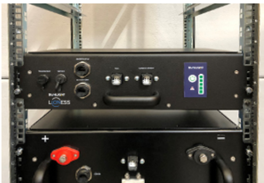
Picture 21b Li.ONESS P.U. installation
