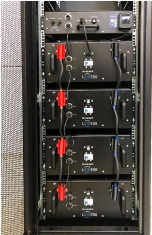
Picture 27 Li.ONESS system, CAN communication connection
