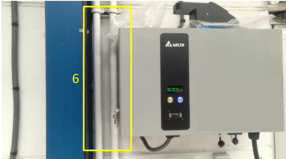
6. Extra pipes or tubes on left side
